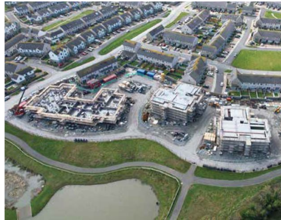
Social housing under construction in Swords
